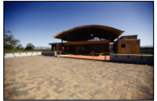
New winery building at Litton Estate
